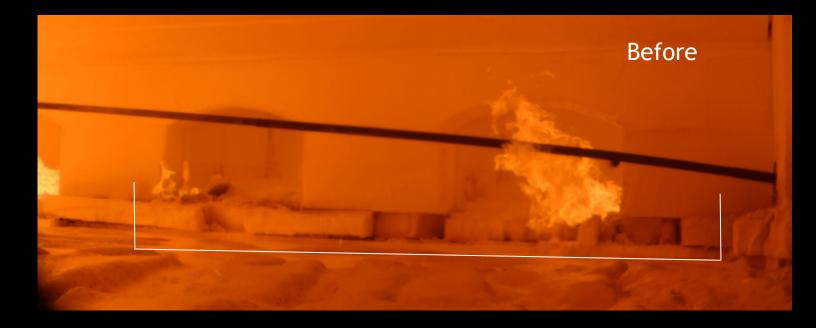
Deteriorated tuck line before and after ceramic welding was conducted.
