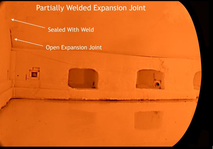
High-Temperature Imaging Our High Temperature Imaging System permits before and after pictures to document furnace changes.
